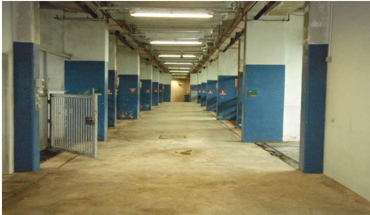
Figure 15: Existing double storey stables
