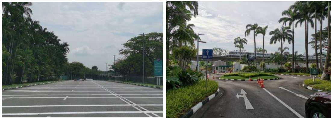
Figure 27: Existing main gantry access from Turf Club Ave (left) and VIP access from Woodlands Rd (right)
