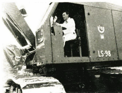
One of the five 32-ton Link-Belt LS-98 excavators bought by Laing Pipelines.
