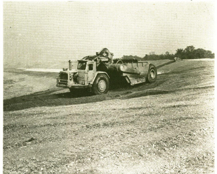
Fig. 7. Caterpillar 631B placing ballast in the embankment
