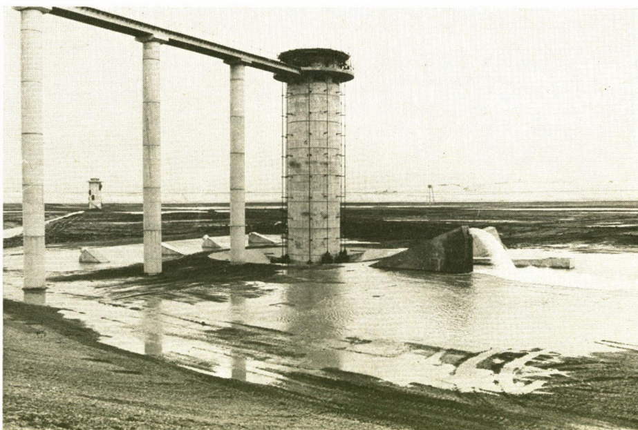
Fig. 1. A 600mm inlet jet in action during the reservoir's first filling in January 1975
