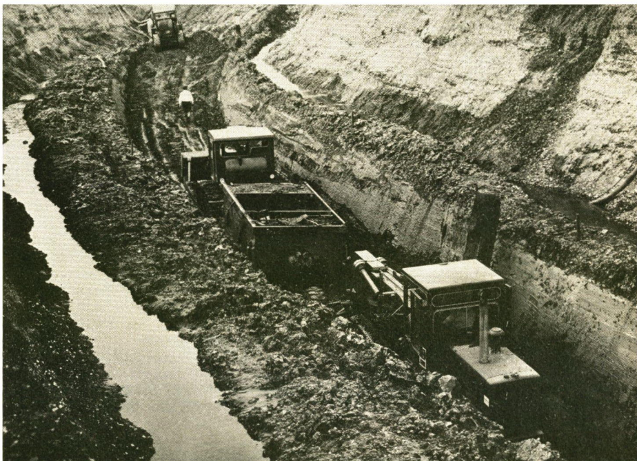
Fig. 5. Compacting the clay in the cut-off trench, showing the 20 ton Albaret roller towed by a D6 and the 14E grader with angled blade forming the battered side of the trench
