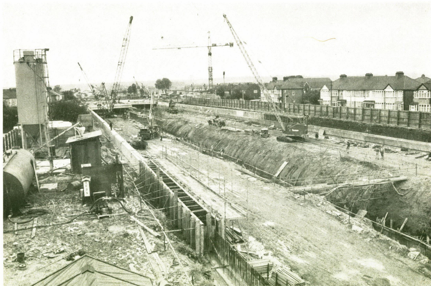
Fig. 1. Construction work in progress for the cut-and-cover M25 Holmesdale tunnel at Waltham Cross. View shows the two diaphragm walls completed either side of the dual carriageways, and the excavation along the line of the central axis
