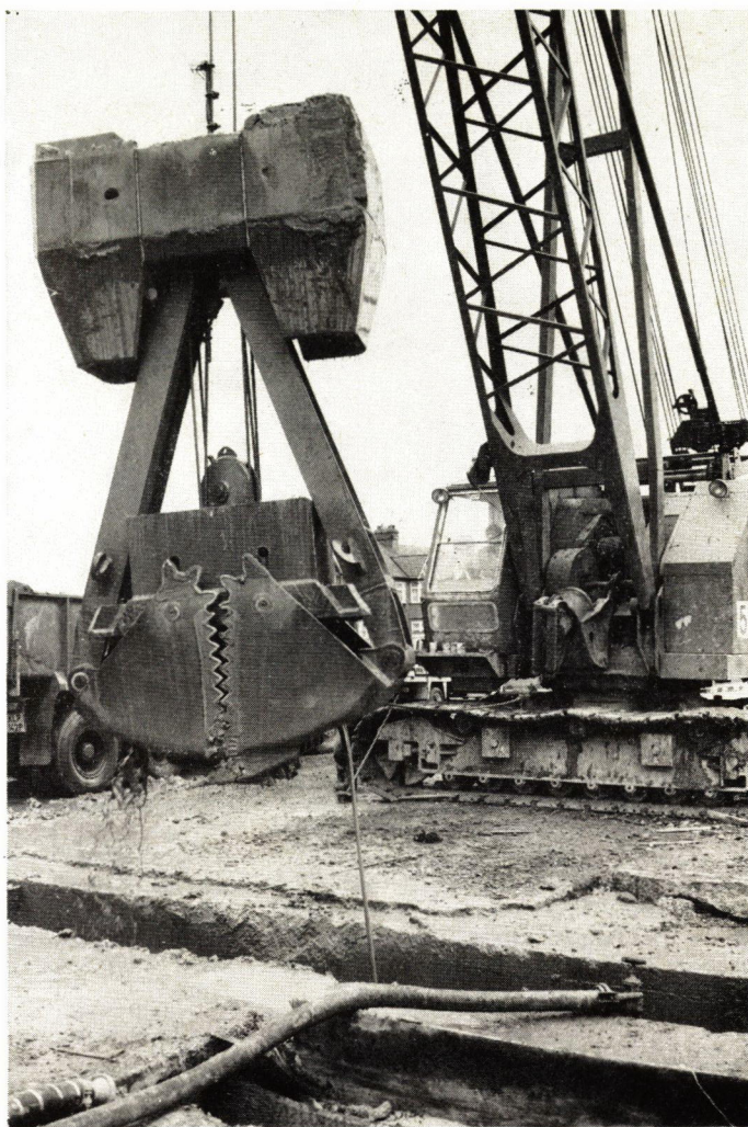
Fig. 7. Excavating for one of the last diaphragm wall panels (across the A1010 Hertford road)
