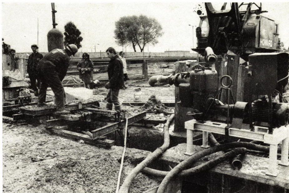
Fig. 8. Panel concreting nearing completion, with bentonite slurry handling pump on the right
