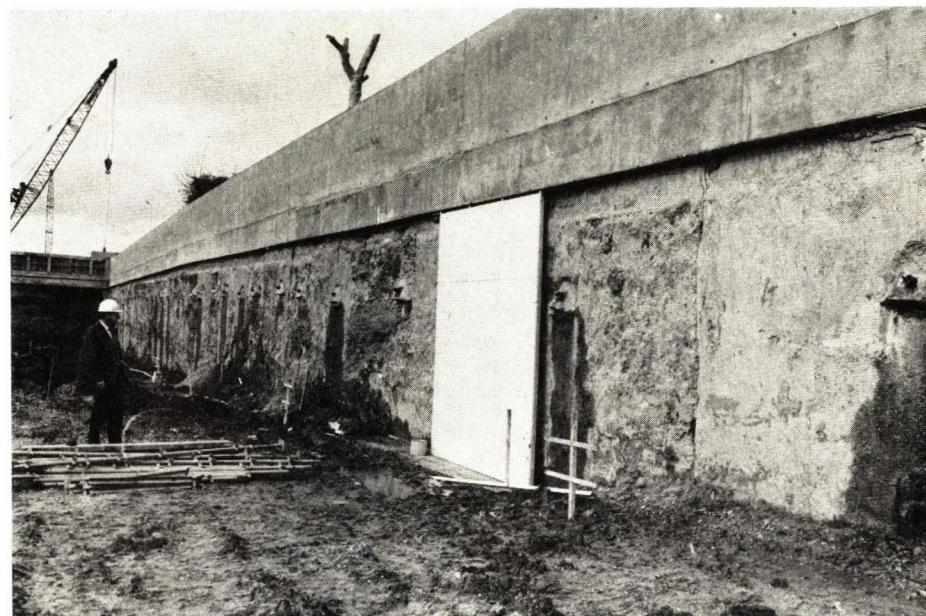
Fig. 9. Section of exposed diaphragm wall to the east of the Holmesdale tunnel, showing a trial panel of cladding material
