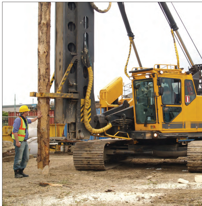
Figure 6: Pile driving trials at a site near Middlesbrough
