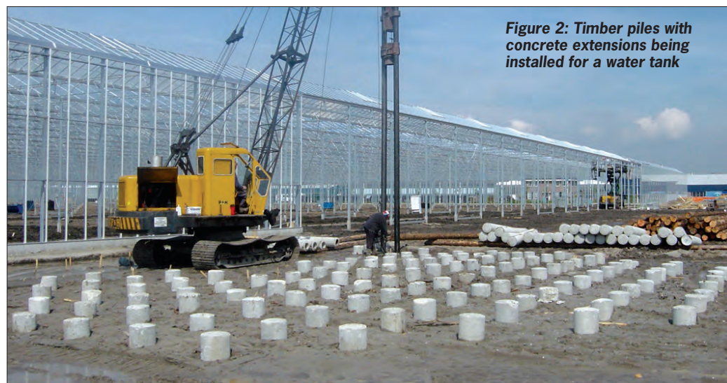
Figure 1: Timber piles with concrete extensions
