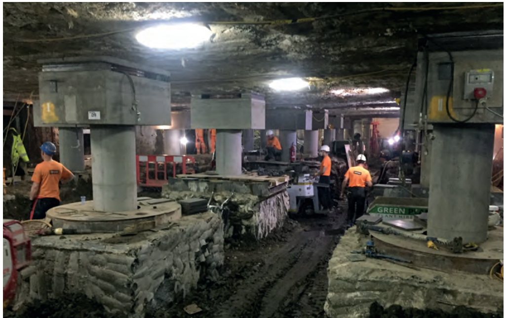
Excavating basement level one revealed the underside of the 1929 reinforced concrete raft
