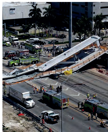
The bridge collapsed onto a busy road
